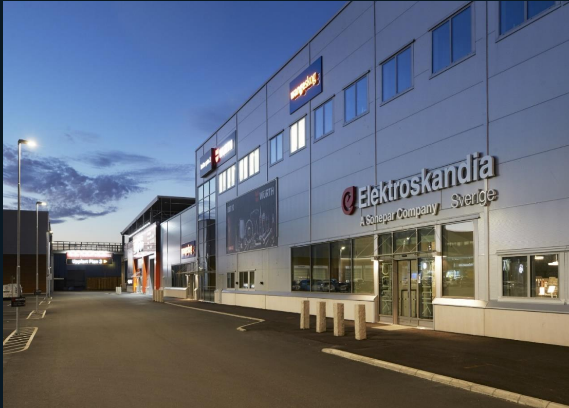
Backa, Gothenburg. New construction of Pro Stop Backa, a specialist retail area in Gothenburg, where K-Bygg, Elektroskandia, Wangeskogs, Würth and Din Bil have moved in.
