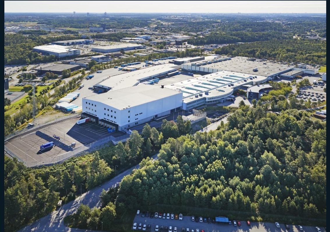
Veddesta 2:79, Järfälla, Stockholm. New construction of an environmentally profiled three-storey warehouse and refurbishment for MTAB in Veddesta, Stockholm
